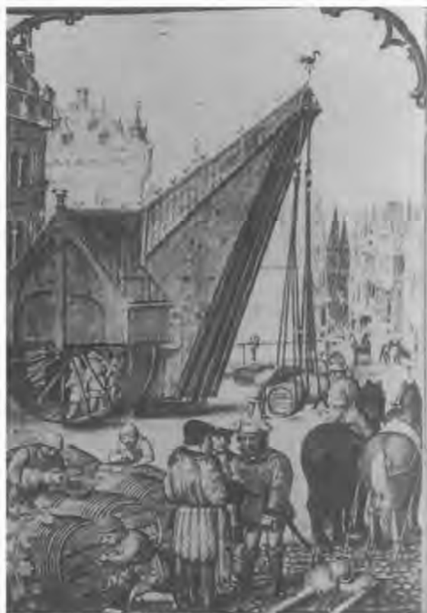
Barge, crane, and canal transshipment of wine. Kranenplatz, Bruges, Hours by Simon Bening. Munich, Bayerische Staatsbibliothek Clm. 23638, fol. 1-1v, 1530.
